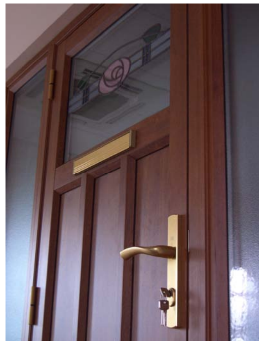
Installed Oak door with side screens
